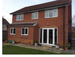
Photo from rear garden (South side)
